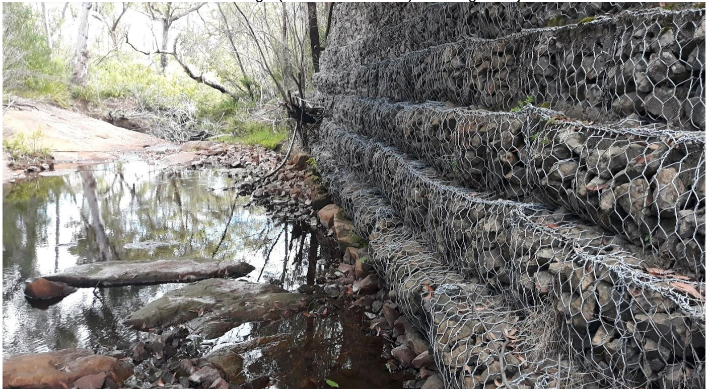
Photo 6: Gabion wall under the bridge (eastern abutment) showing Boolijah Creek
