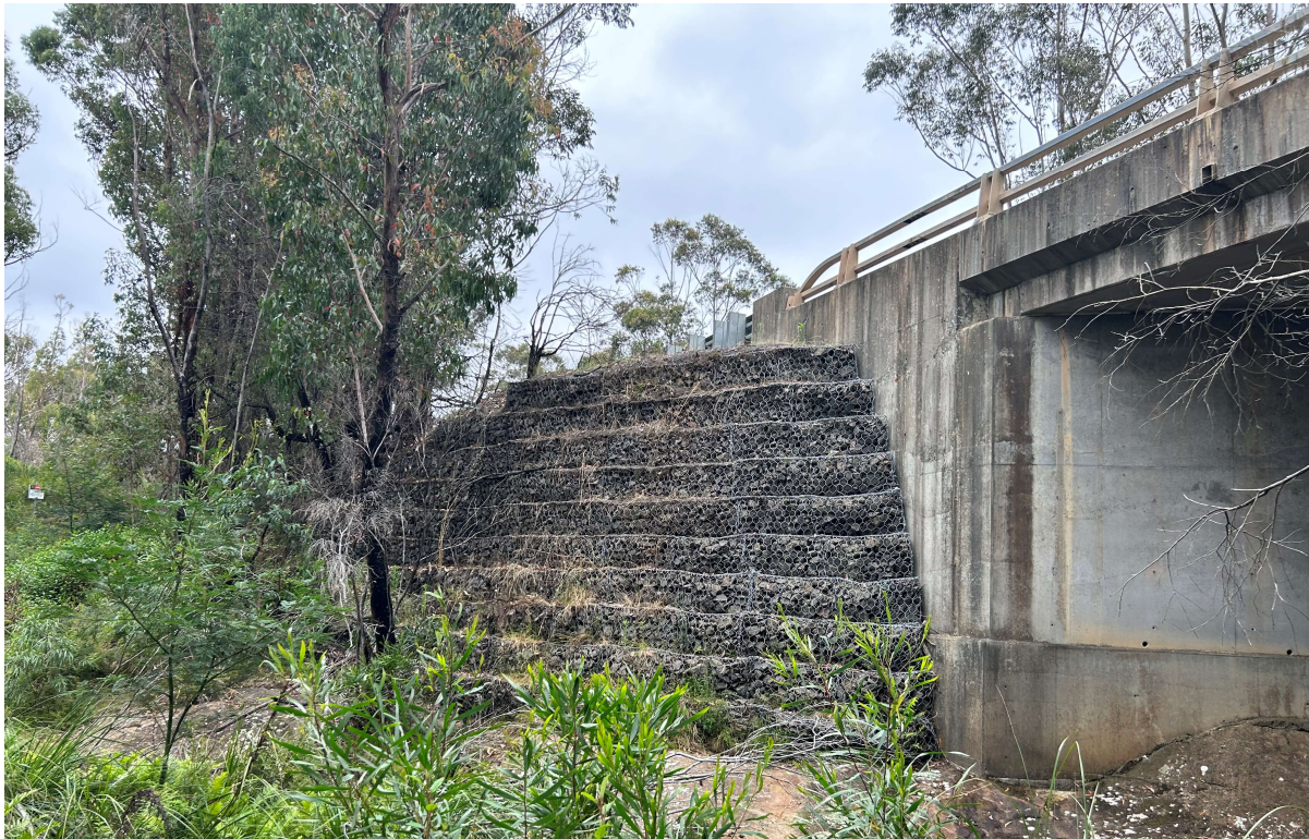
Figure 1 Southwest bridge abutment
