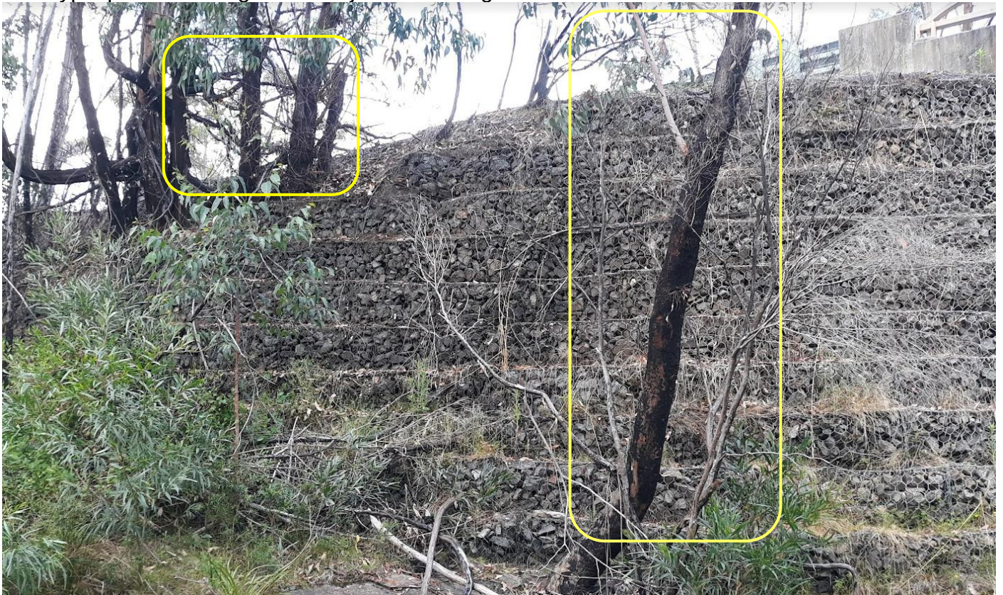
Photo 4: Gabion wall on the south-western wing of the bridge. Showing approx four to five Eucalypts plus other vegetation adjacent to the gabion which will be removed.
