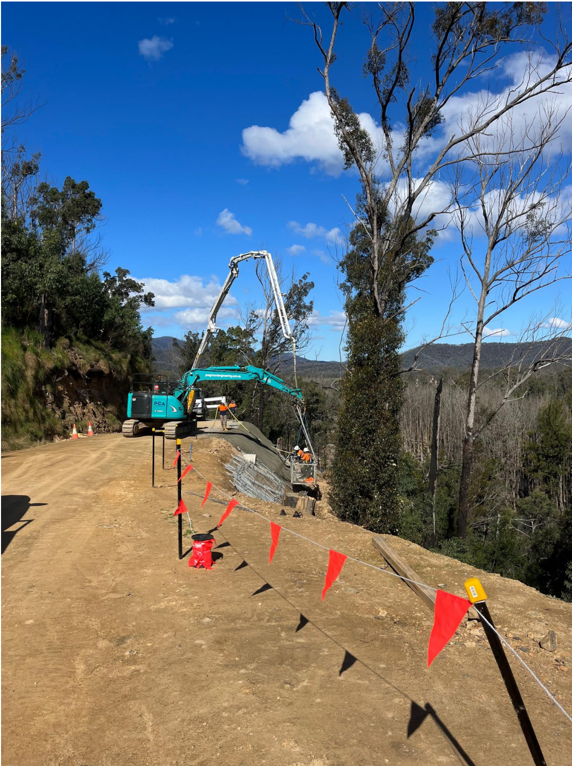
Example pic from a similar PCA project (Araluen Rd NSW, 2022)
