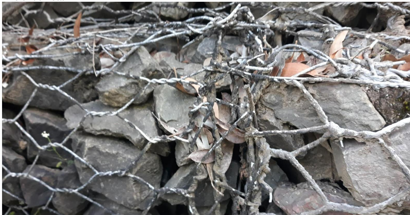
Photo 2: Example of fire damage to wire netting on gabion with plastic coating melted exposing wire underneath
