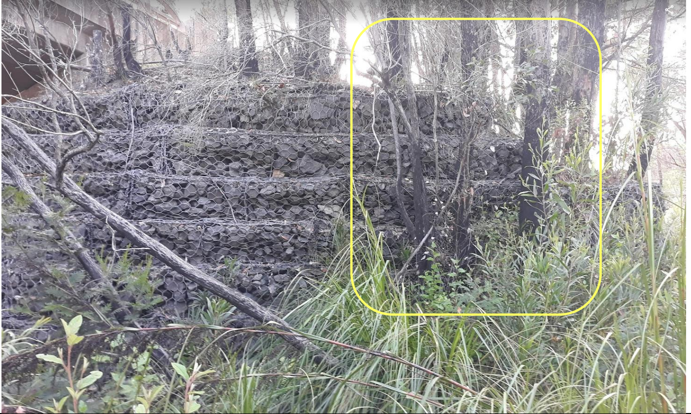
Photo 4: Gabion wall on the south-western wing of the bridge. Showing approx four to five Eucalypts plus other vegetation adjacent to the gabion which will be removed.
